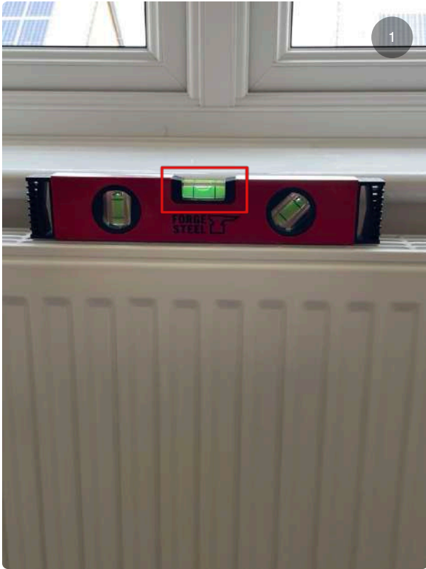
Snag 1 Master Bedroom Radiator not level
